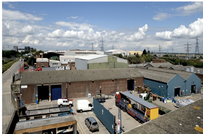
A view of the work-shop users. One of the first tasks was to underground the huge electricity pylons seen in the distance. This is expensive. It also 'sterilises' the ground for the huge high-tension cables can not be built-over.
