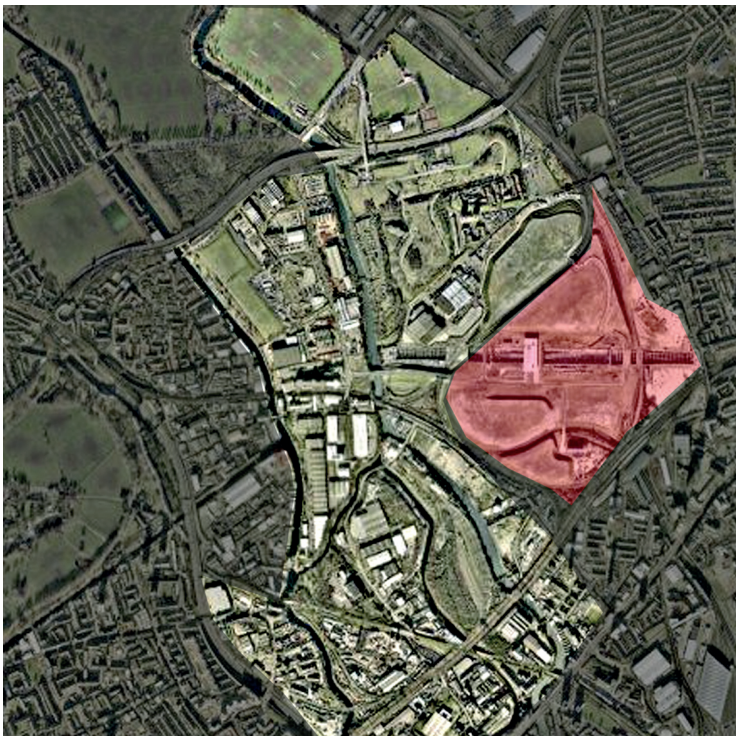
An aerial of the site shows, in pink, the rail marshalling area all cleared, and ready for construction of the commercial surroundings to Stratford Eurostar. The factories remain. A last testament to the 1947 project, reported in Lecture Three: 'The End of Urbanity' to rid British cities of 'workers'.
